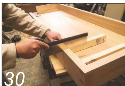
30 The apron is notched for the mechanism...
